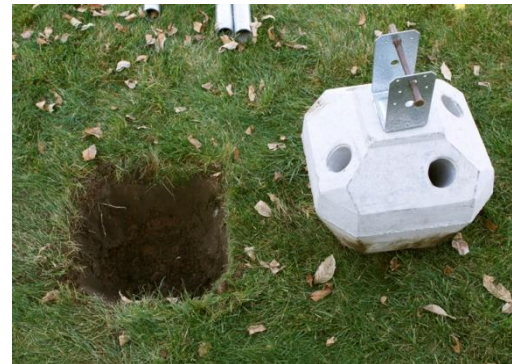
Figure 5. Tapered Hole for Concrete Head
