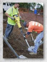
The patented Diamond Pier Foundation combines high-strength pre-cast concrete heads with 4 galvanized steel bearing pins. The pins slide through guides in the concrete head and are driven into penetrable native soil to create a strong, efficient, low-impact foundation.
