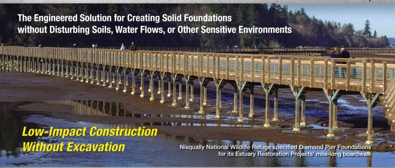
Diamond Pier Foundations are suitable for **Low-Impact Construction** in parks, preserves, campuses and public spaces. The system's non-destructive technology allows boardwalks, platforms, decks, overlooks, pavilions, bridges and stairways to be built with minimal site disturbance reducing erosion and site compaction and preserving the integrity of existing soils, native vegetation and the natural flow of ground water.
