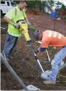
The patented Diamond Pier Foundation combines high-strength pre-cast concrete heads with 4 galvanized steel bearing pins. The pins slide through guides in the concrete head and are driven into penetrable native soil to create a strong, efficient, low-impact foundation.
