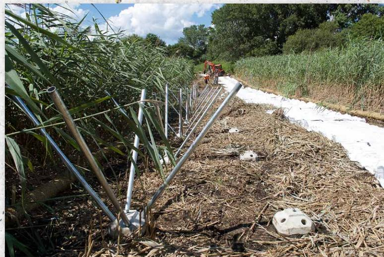
Engineered Diamond Pier Foundations fit into any low impact design strategy, bringing an environmental solution to a wide variety of construction sites.
