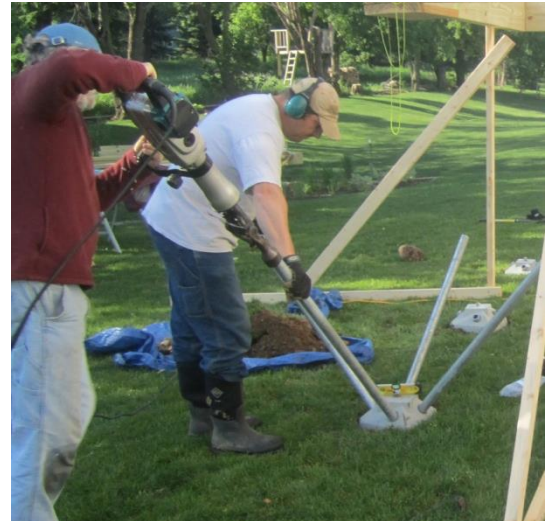
Figure 7. Driving Pins with Auto-hammer and Pin Driving Bit
