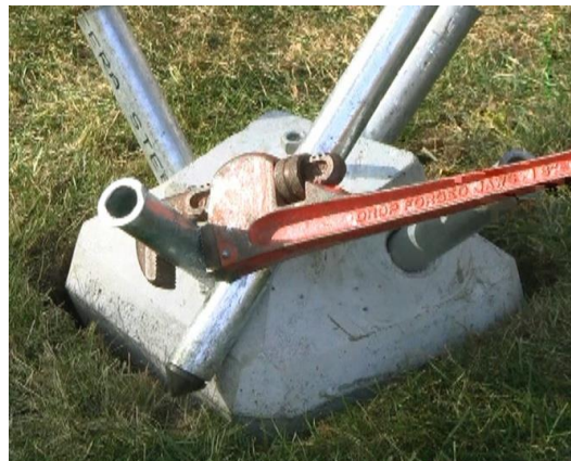
Figure 8. Jacking Method for Pin Removal
