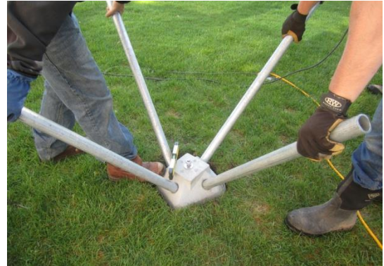
Figure 6. Setting Pins and Leveling Concrete Head
