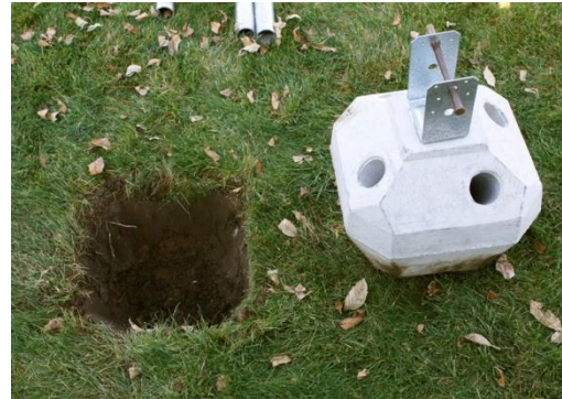
Figure 5. Tapered Hole for Concrete Head
