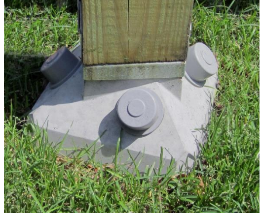
Figure 7. Completed Installation with Pin Caps
