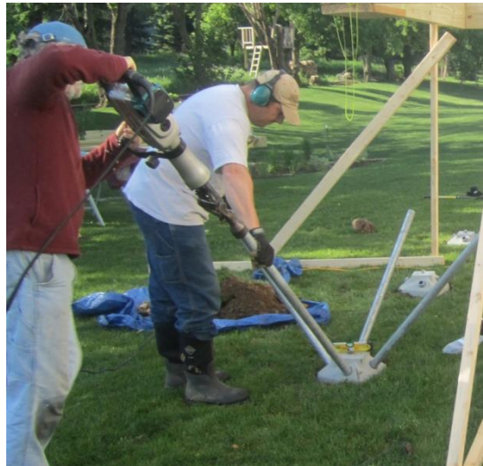
Figure 5. Driving Pins with Auto-hammer and Pin Driving Bit
