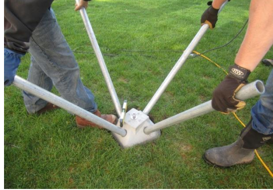
Figure 4. Setting Pins and Leveling Pier
