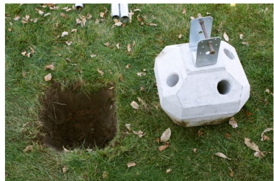
Figure 3. Tapered Hole for Concrete Head
