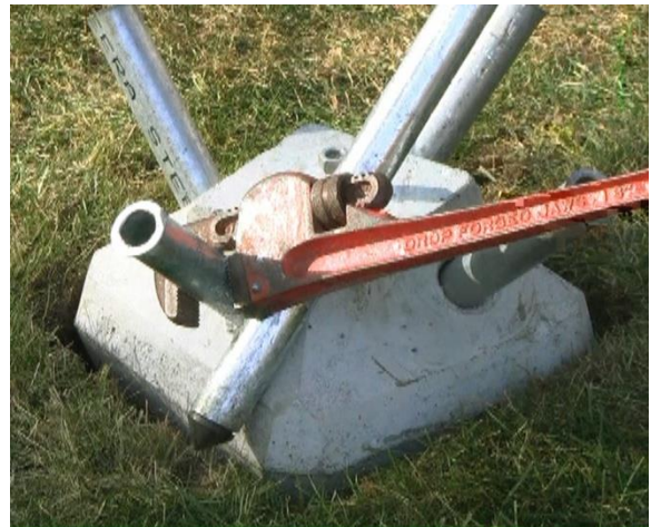
Figure 6. Jacking Method for Pin Removal
